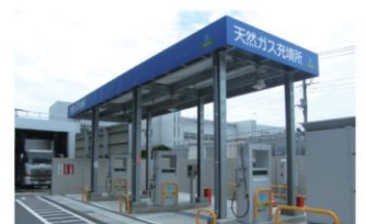
Natural gas station of a logistics company
